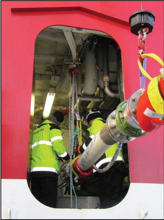
Connecting 6" Cryogenic Coupler and Breakaway
